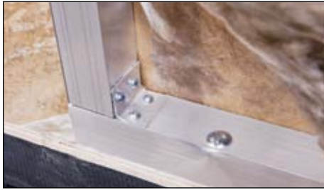
All aluminum sills and wall studs are mechanically joined and the aluminum sill tubing is fully reinforced internally with wood, providing greater strength and stability when it is "bolted-through", never screwed, to the sub-floor structure and the steel frame below.
