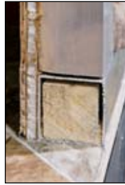
All aluminum sills and wall studs are mechanically joined and the aluminum sill tubing is fully reinforced internally with wood, providing greater strength and stability when it is "bolted-through", never screwed, to the sub-floor structure and the steel frame below.
