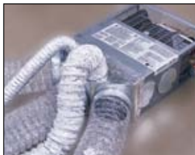
High density wool insulation blankets the underbelly frame spaces and the flooring assembly, to provide added protection for the water systems. Perimeter heating features 6" ducts and custom plenum with 5-duct heating.
